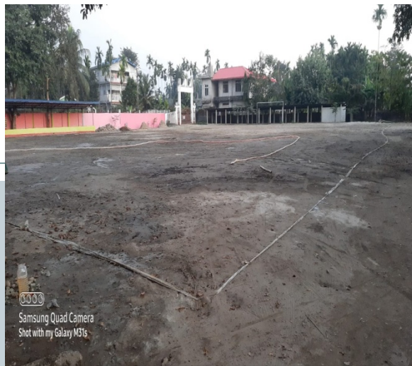
Play Ground Renovation
